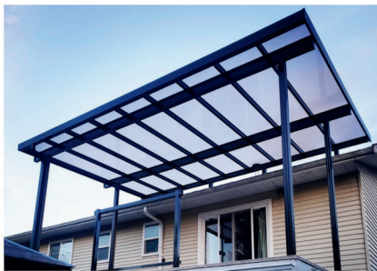
ON TOP OF ROOF
